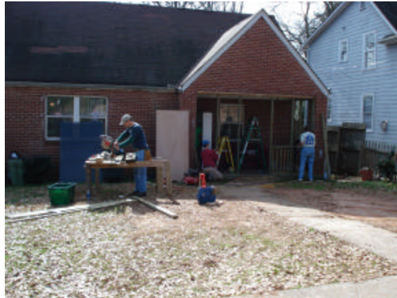
Volunteer workers rebuild the Hill family's front porch.
